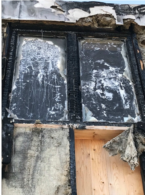
Figure 3.35 Fireproof window on facade 1-1 after the test
