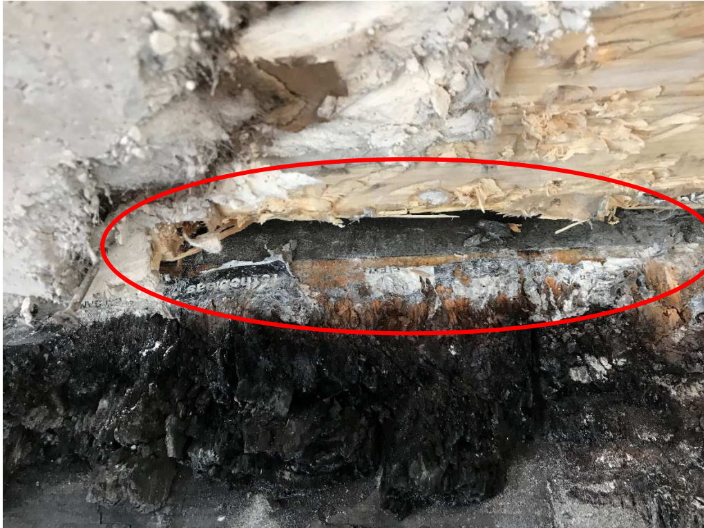
Figure 3.20 Deconstructed wall-floor joint meant for larger scale buildings. No expansion of intumescent tape has happened
