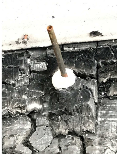
Figure 3.29 Expanded intumescent material around the tube
