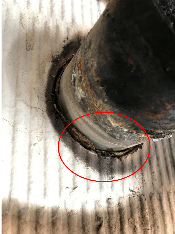
Figure 3.27 Acrylic material used to seal the hole
