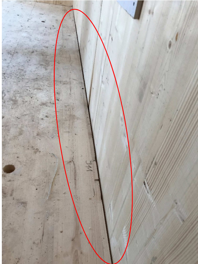
Figure 3.17 J11's location as seen from the upper floor. Visual inspection shows the joint to have worked perfectly due to no observable smoke or heat damage
