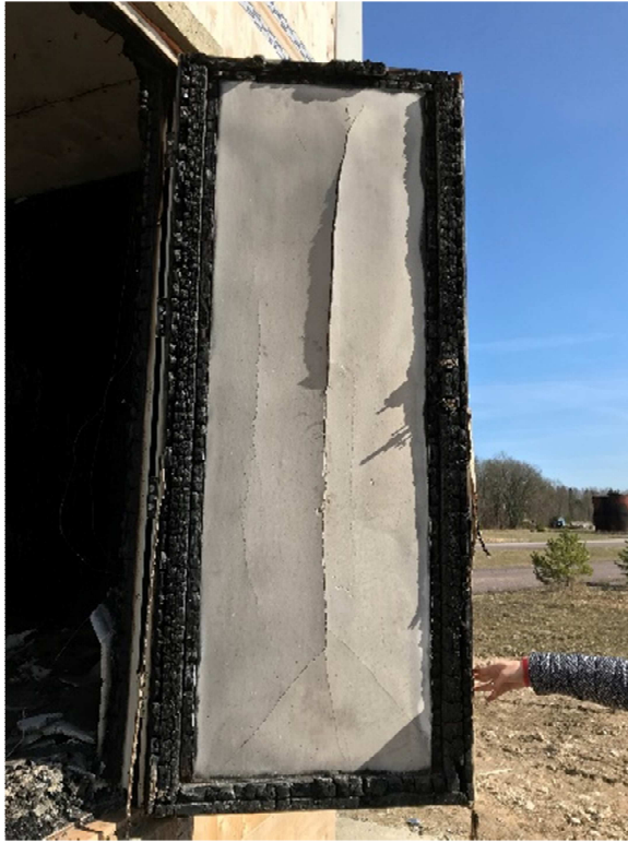
Figure 3.37 Inner face of the door after the test
