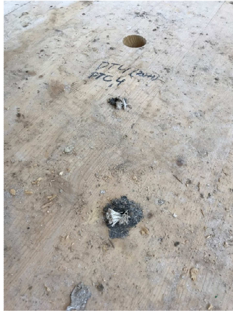
Figure 3.30 Graphite-based material in the ceiling penetrations as seen from the upper floor
